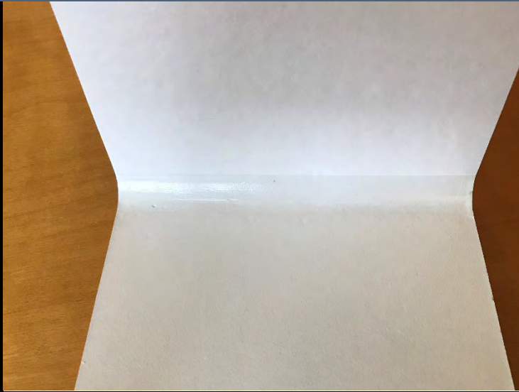
Textured Epoxy Toilet Flooring
